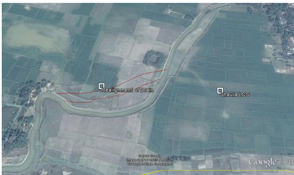
Figure 4.2: Rainwater Drain in the Proposed Sheola Land Port Area
